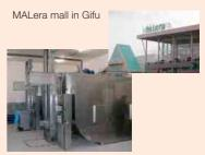
One of the largest biodegrading waste processors is installed at the MALera mall in Gifu, Japan. This system can process 750kg of garbage a day.
