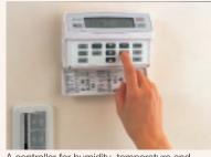
A controller for humidity, temperature and ventilation
